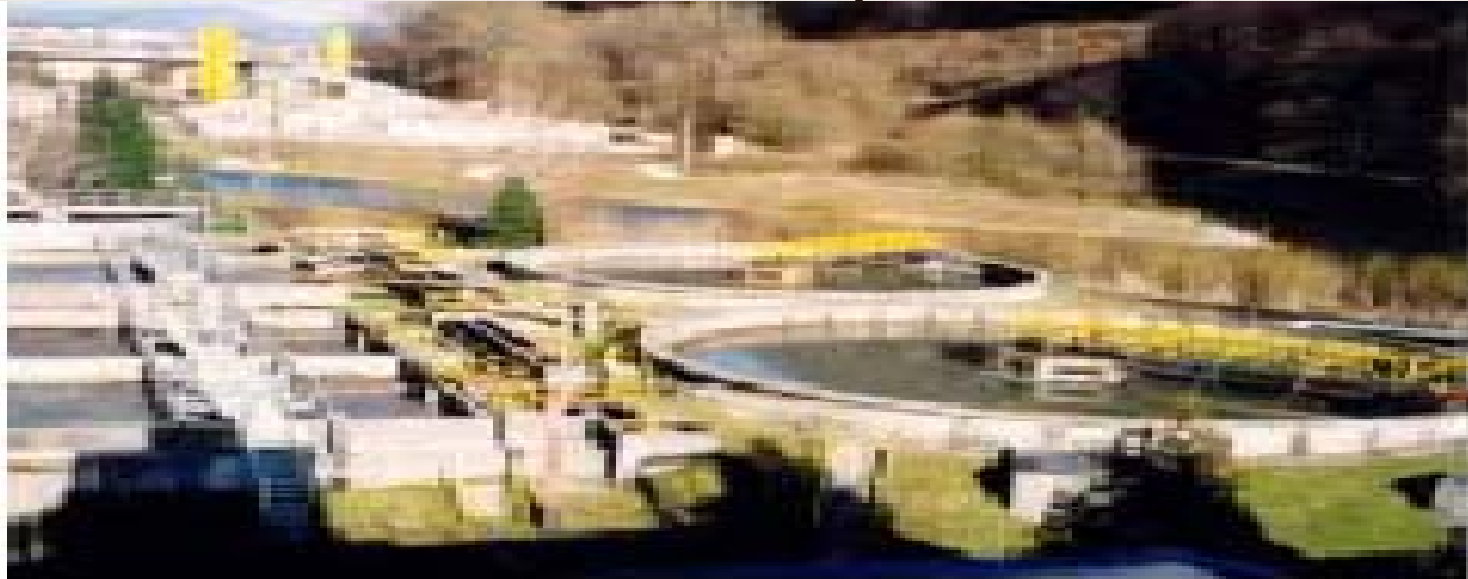
Waste Water Treatment Plant – Poland
